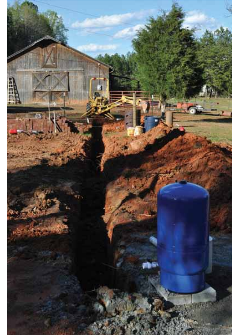
Buster digs a water line trench
